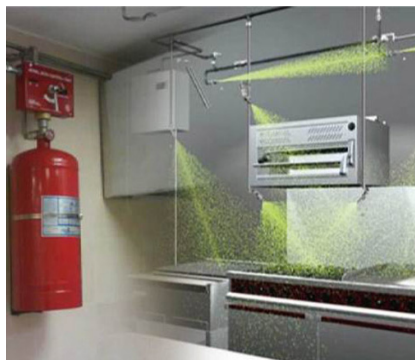
Wet Chemical Kitchen Hood System
